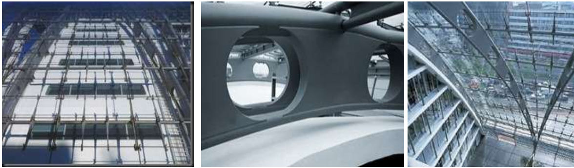
Figure 2.0.1.8. Berliner Bogen Office Building
