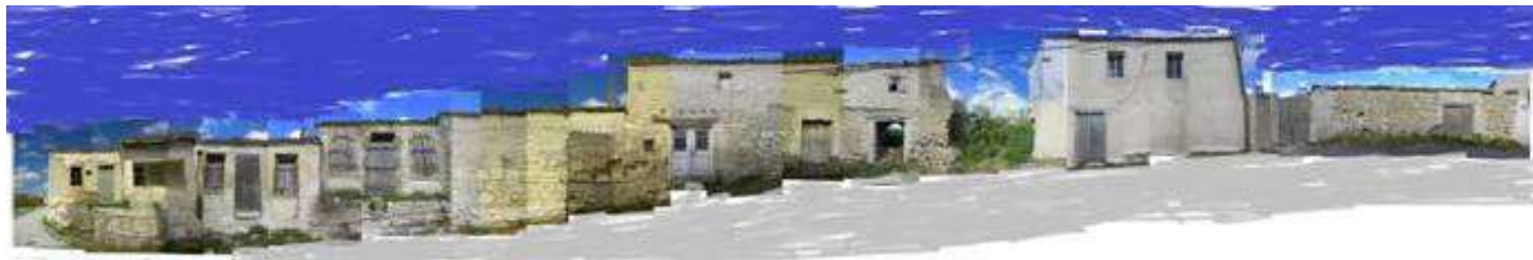
Figure 4.3.1: Veli Usta Street From West
